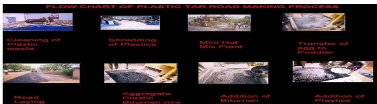
Figure 5: industrial waste Plastic Tar making process
